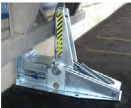
**Blue Giant hydraulic vehicle restraints** hold trucks securely at the loading dock, improving safety levels during cargo handling operations.
